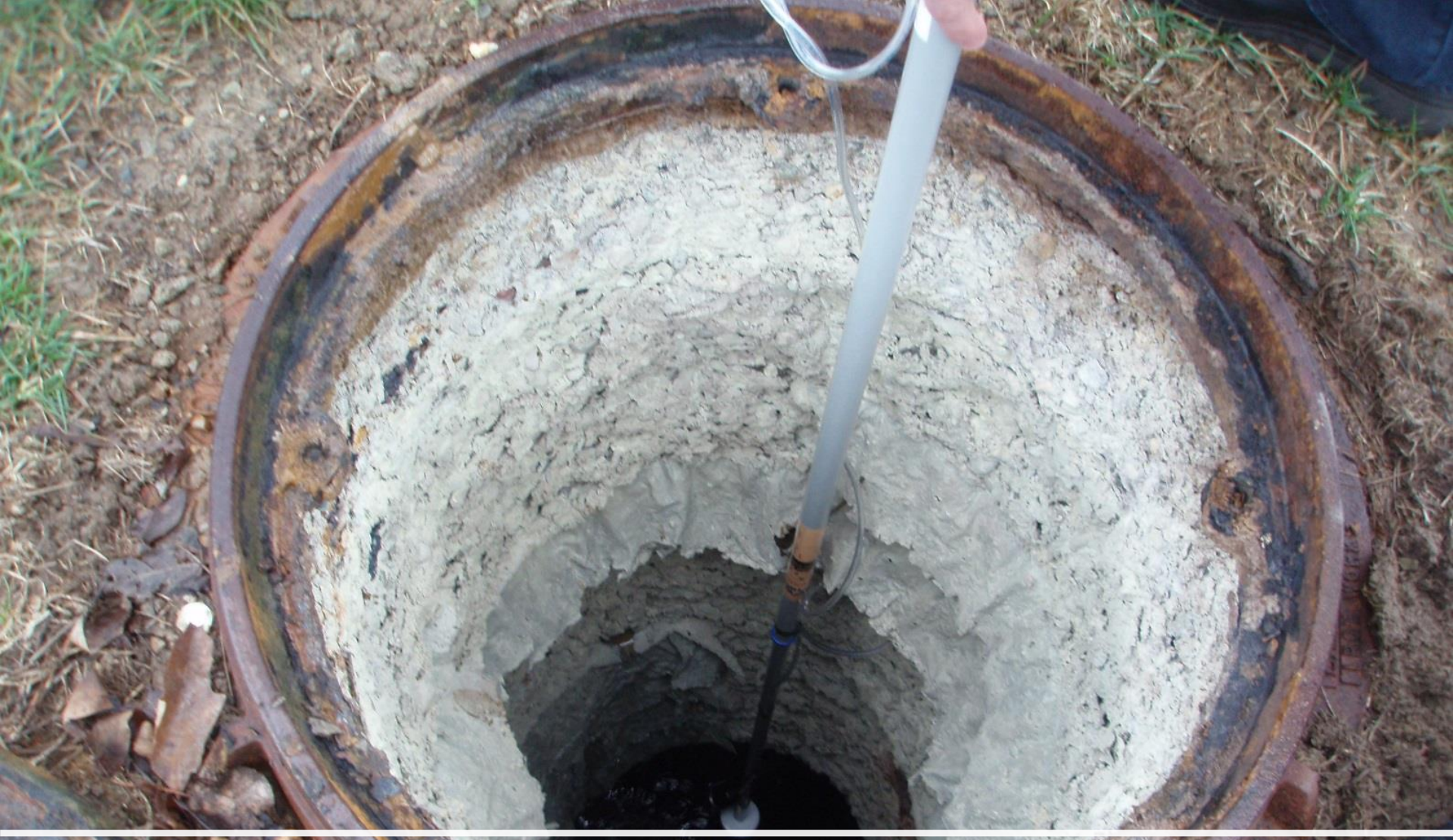
Concrete Corrosion
