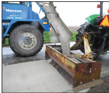
Hanson supplying the ready mix grout into the spreader box
